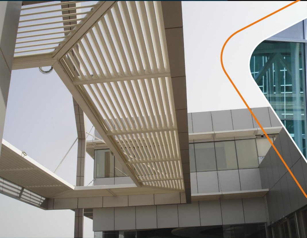
Pre-fabricated sun shades and louvers.
