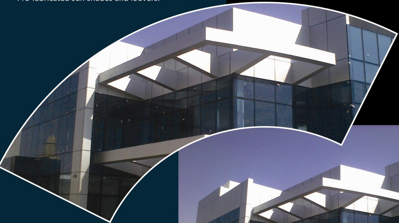
Pre-fabricated sun shades and louvers.
